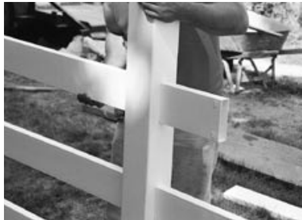
Rails are threaded through the pre-routed posts.
