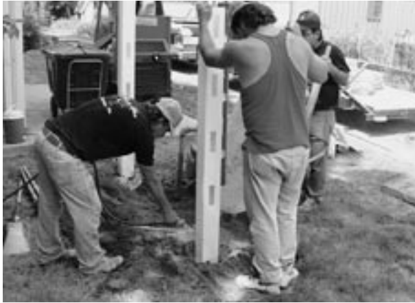
Holes dug, posts aligned and initially tamped in dry cement, water is being added to set the posts.
