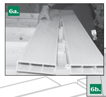
6. (a) Snap the spring forks on the Delrin clips into the outer edge of the second plank and then fit the inside edge onto the outside edge of the first board, utilizing the previously attached Delrin clips. Insert the screws in the outer edge of the next board. (b) Repeat this process with each successive row.
